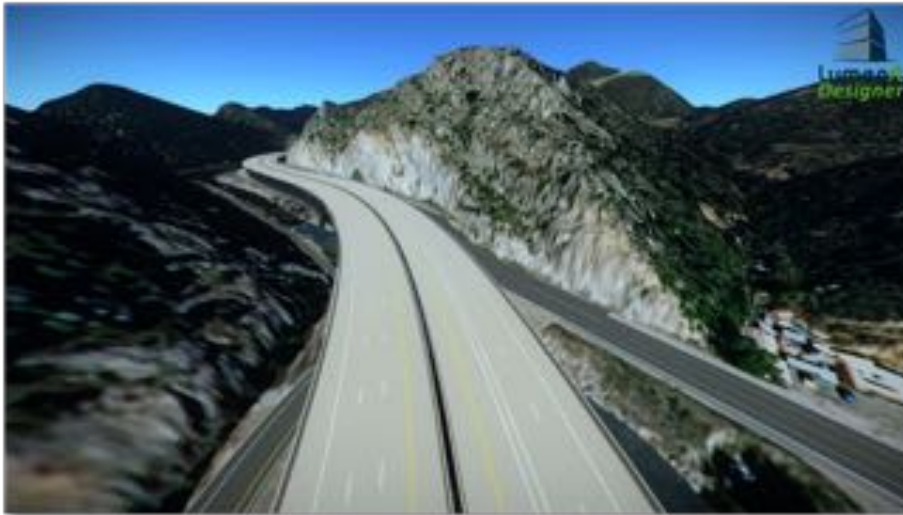
East Portal – Looking West (Figure 4)
