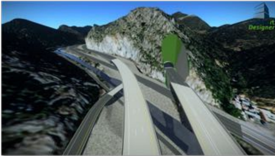
East Portal – Looking West (Figure 1)
